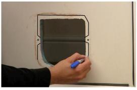
Mark the line out in permanent marker – and proceed to cut along the lines –leaving the screw holes in place as shown.
