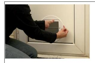
Using the SureFlap mounting adaptor as a guide trace around the circumference of the circular mounting adaptor.
