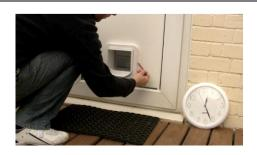
You will need to cut a larger hole in your door – leaving a gap of 2-3cm between the tunnel of the SureFlap and the metal in your door.
