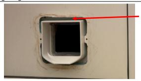
The hole will then look like this and you can retry the installation using your original drilled holes.
